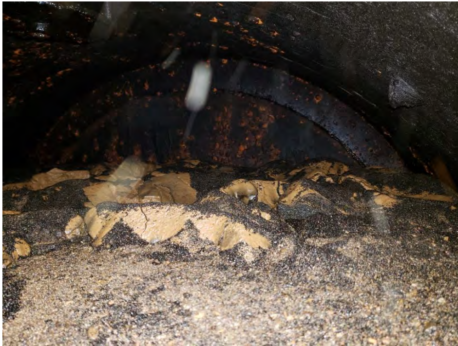
Filter No. 2, Cell 2, Channel Erosion with Surface Silt
