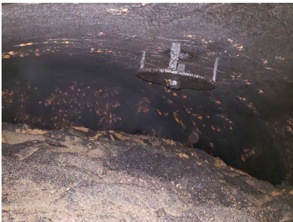
Filter No. 2, Cell 1, Uneven Surface with Mud Balls
