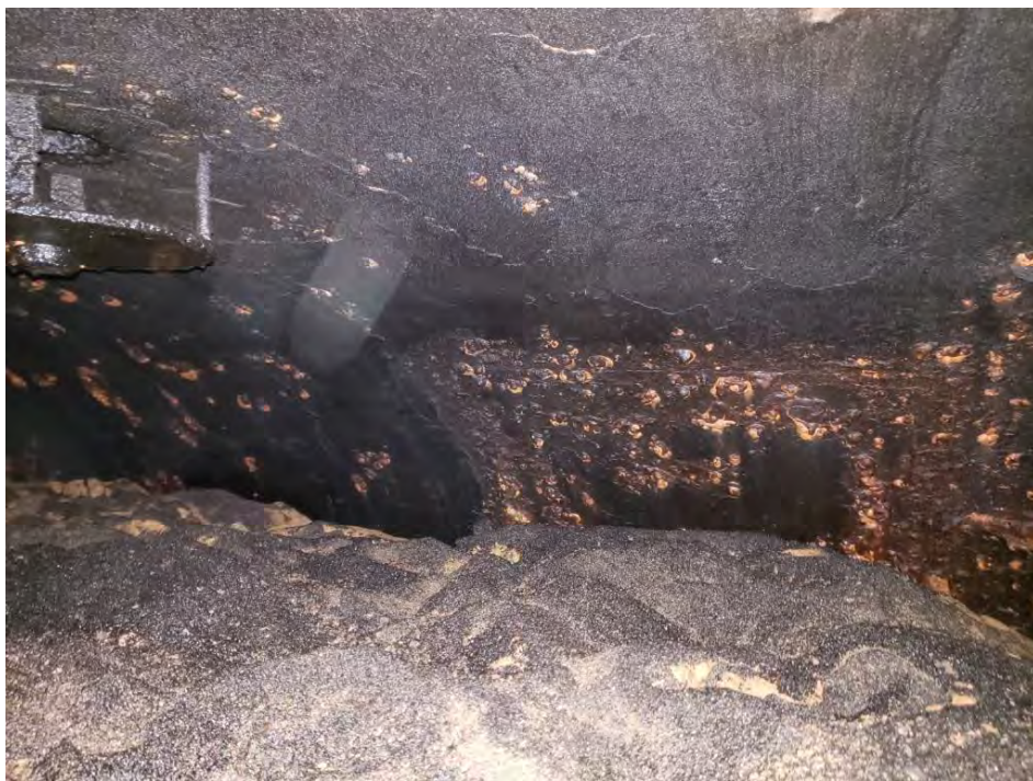
Filter No. 2, Cell 1, Uneven Surface with Some Visible Silt
