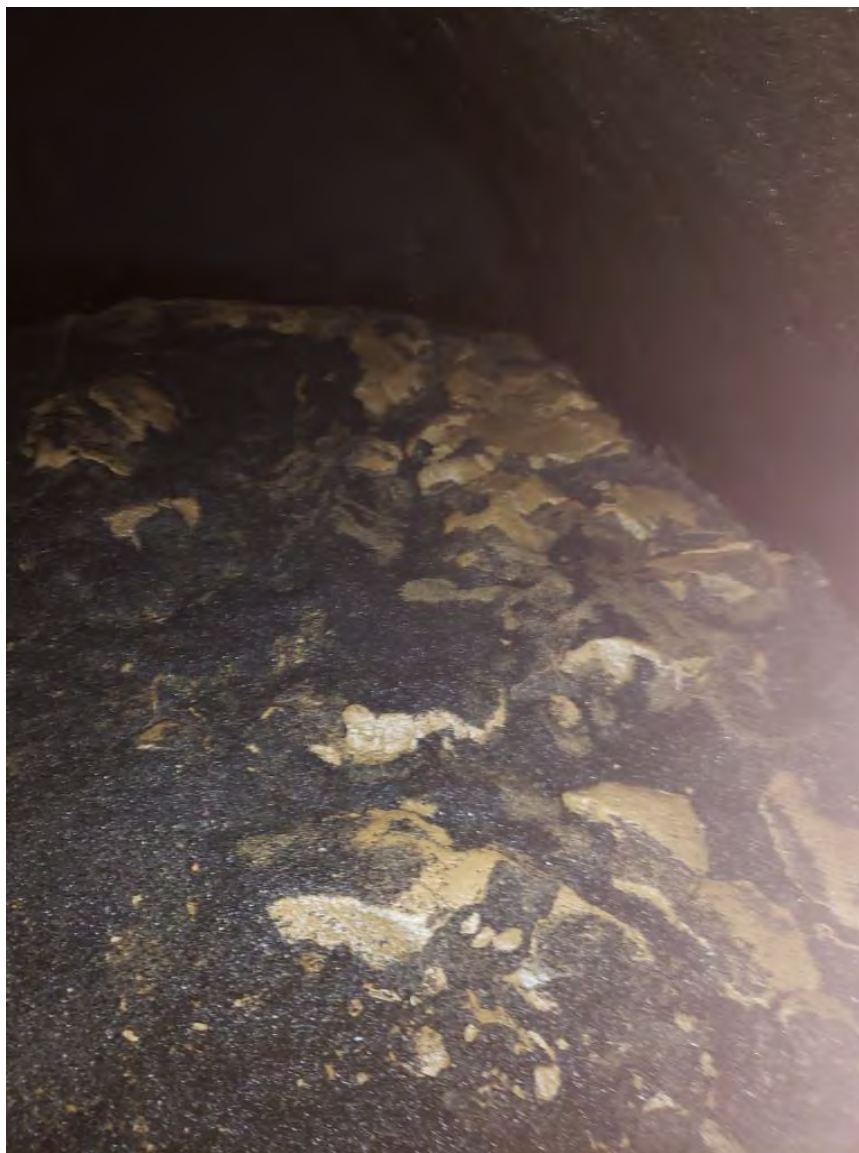
Filter No. 1, Cell 1, Media Surface with Some Sediment Visible
