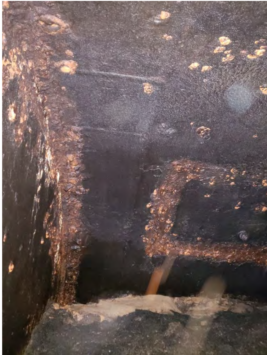
Filter No. 1, Cell 3, Repairs of Baffle Wall Between Cells 2 and 3
