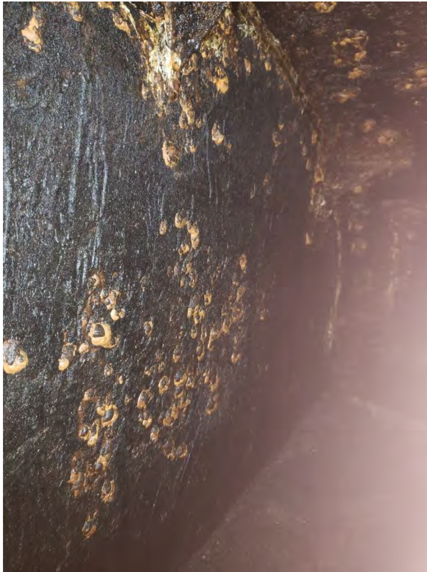
Filter No. 1, Cell 1, Corrosion on Baffle Wall Between Cells 1 and 2
