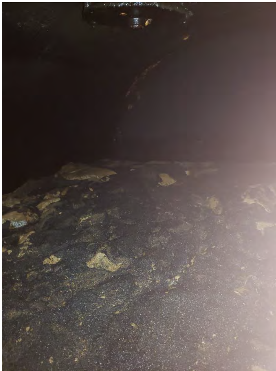
Filter No. 1, Cell 1, Light layer of silt/sediment remained on surface of media.
